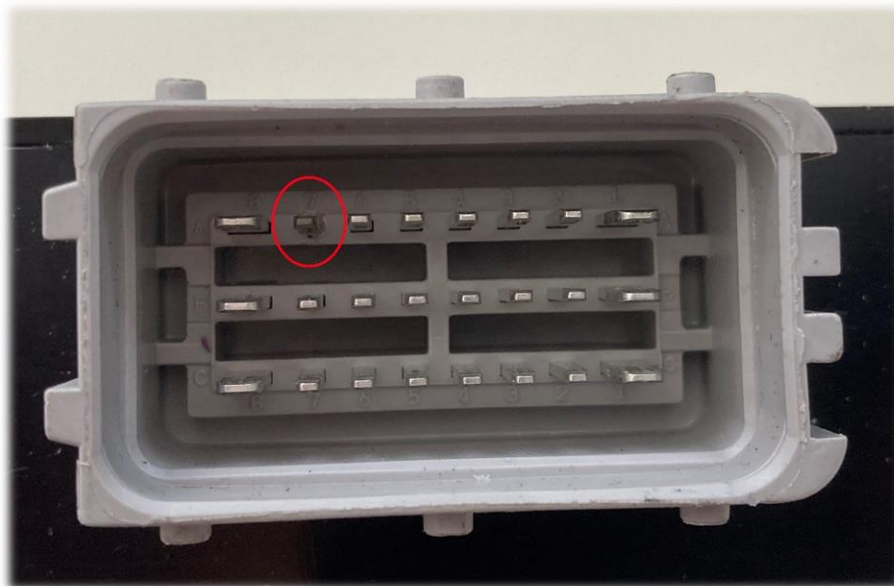
Fig.5: PIN 7A failed, powerbox side.
